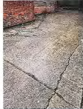
Figure 5: Cracks along the edge of the concrete slabs
