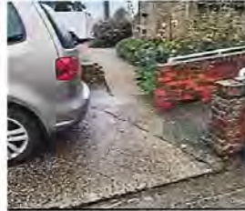
Figure 2: Trip Hazard along Footpath leading to Church Approach
